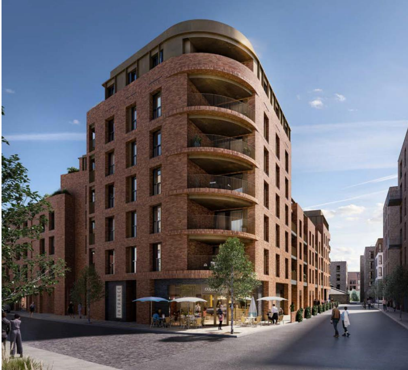
View looking south at northwest corner of proposed building within HRWMF
