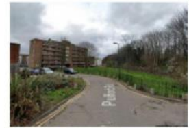
C. Existing view
